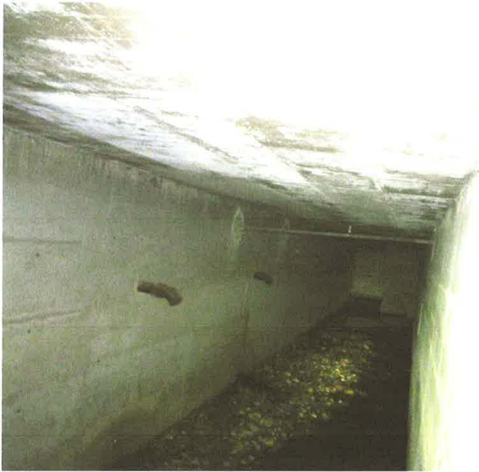
Culvert looking upstream
