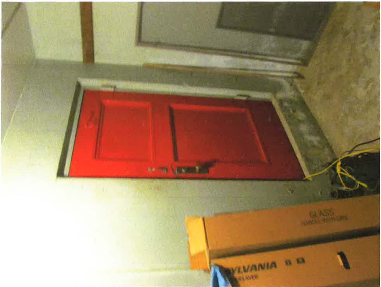
outer door to culvert
