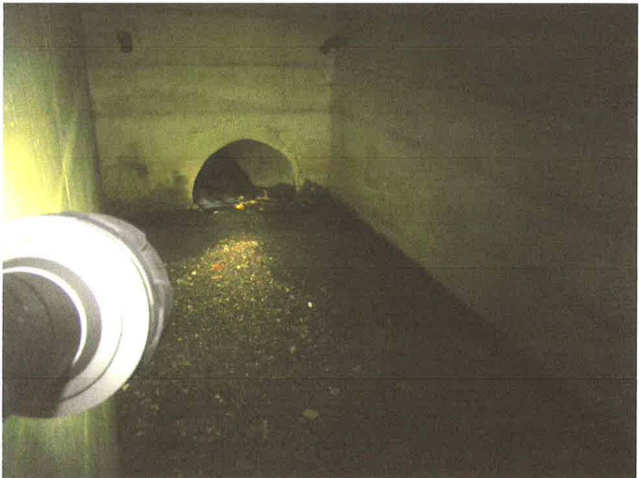
Culvert looking downstream
